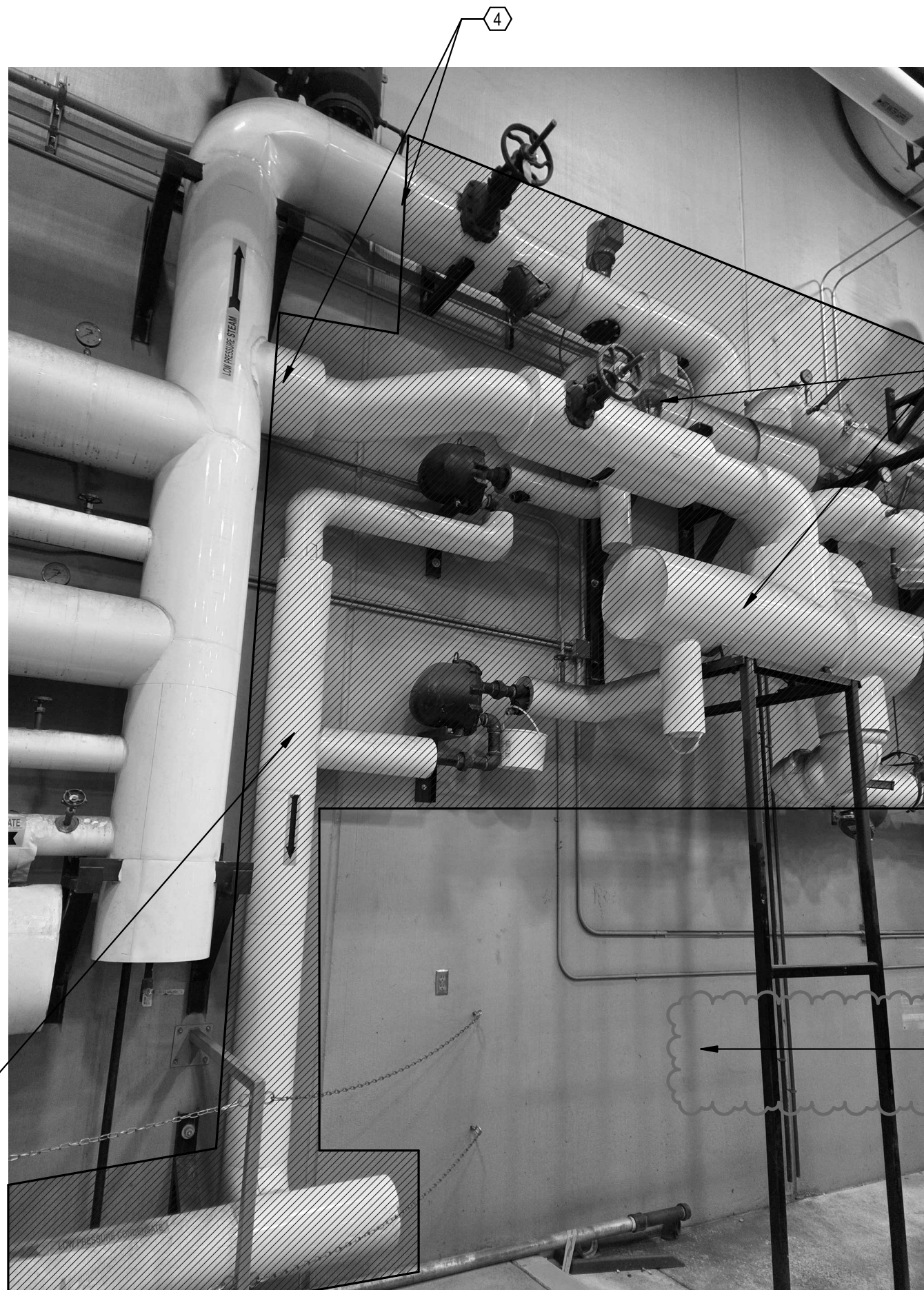
B4 STEAM SYSTEM DEMOLITION 2 MD101/ NO SCALE
