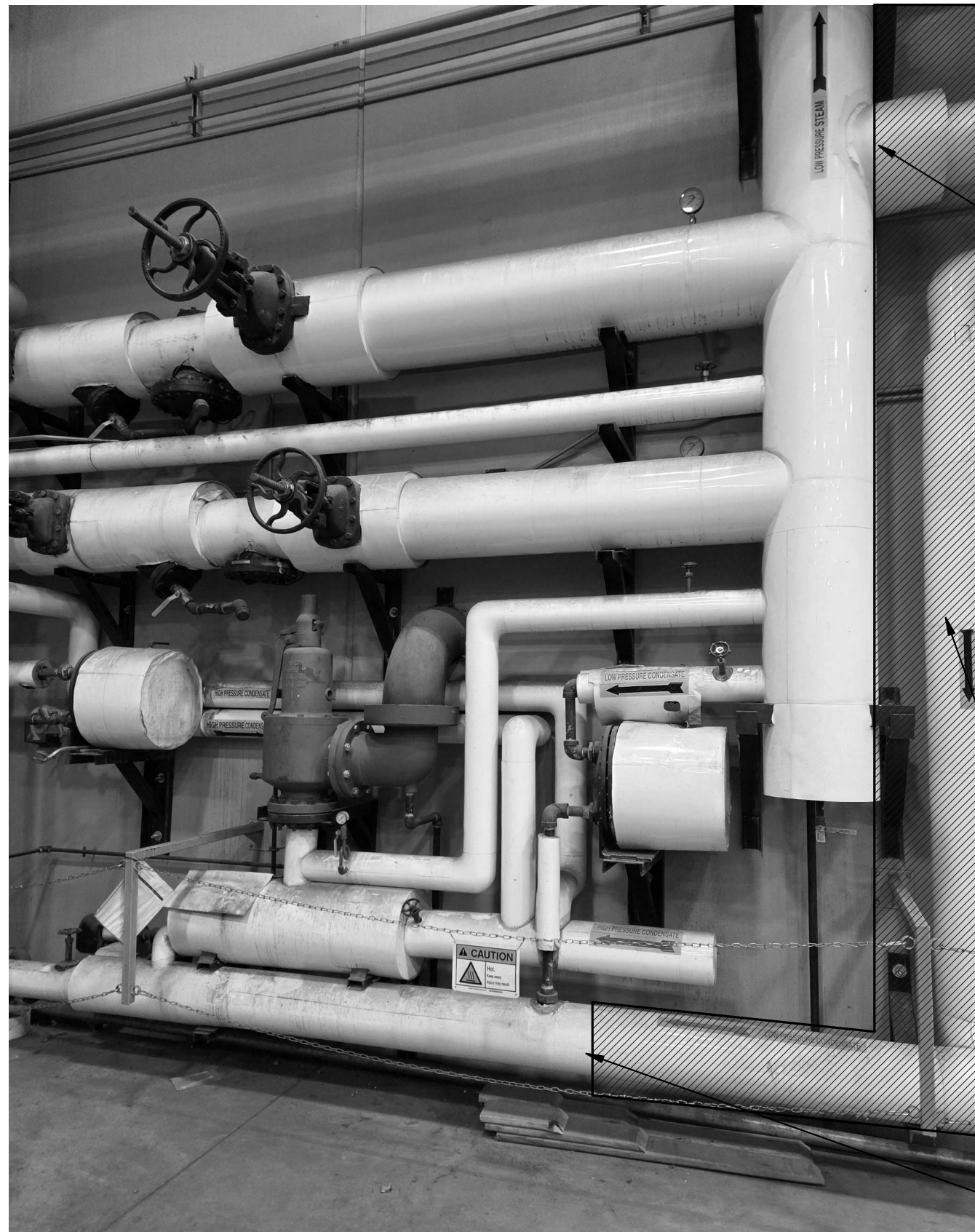
B5 STEAM SYSTEM DEMOLITION 1 MD101/ NO SCALE
